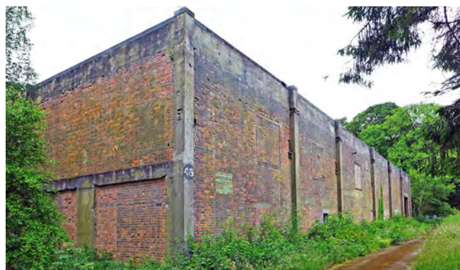
Building 45, originally designated P6 and intended for mustard gas manufacture. Later converted for use by the ‘Tube Alloys’ project to concentrate Uranium 235
